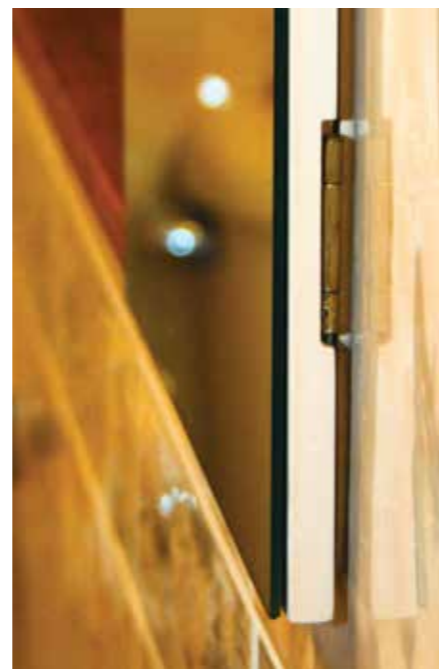
The doors needed to fit neatly against the tiles
