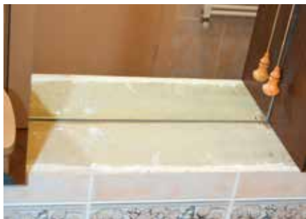
Ready for the sill to cover the exposed tile edges
