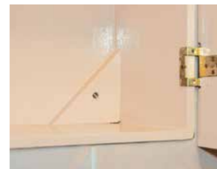
Here you can see the detail of the corner blocks and hinges
