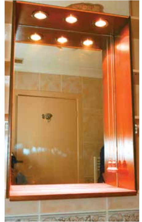
The mirror recess complete with lighting pull cord
