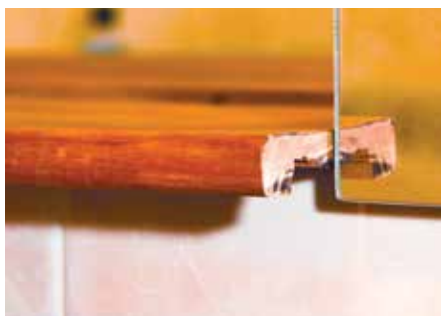
The lipped sill profile; ready to push back to cover the tile edge
